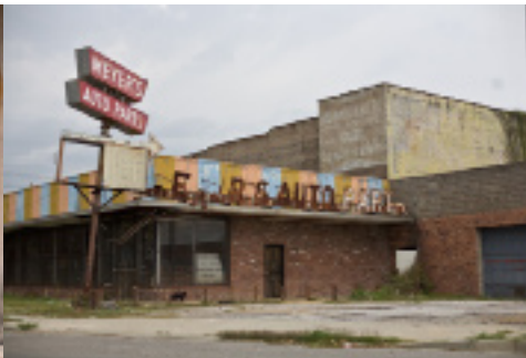
Abandoned retail space in New Orleans, three years after the disaster Katrina.
